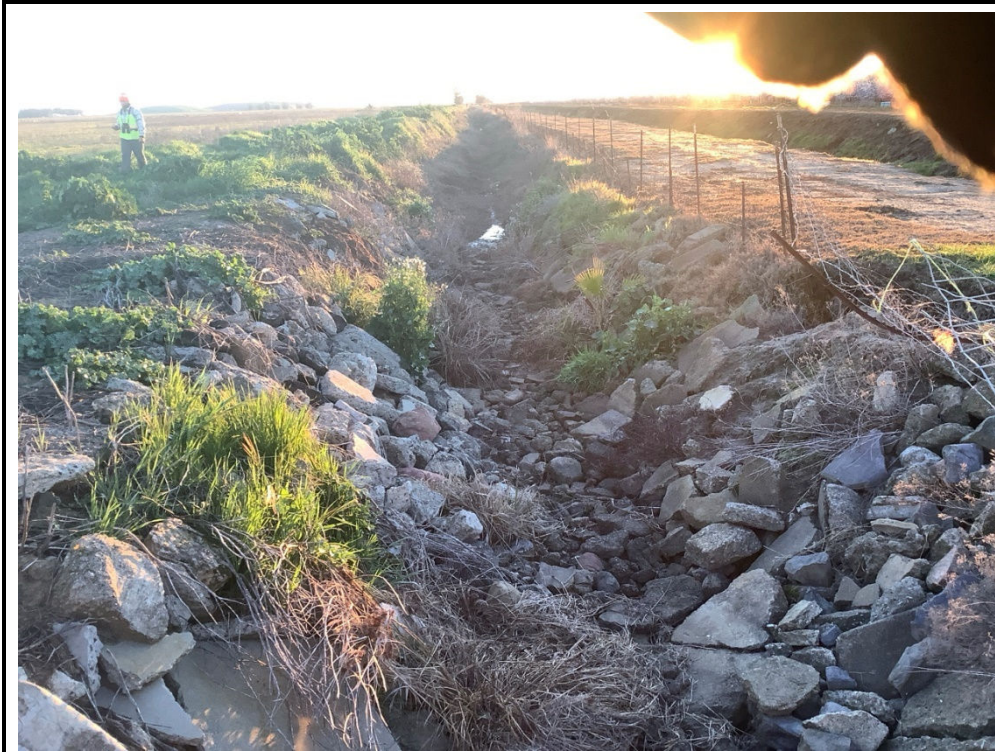
Photograph 5: D-3, facing upstream and east.
